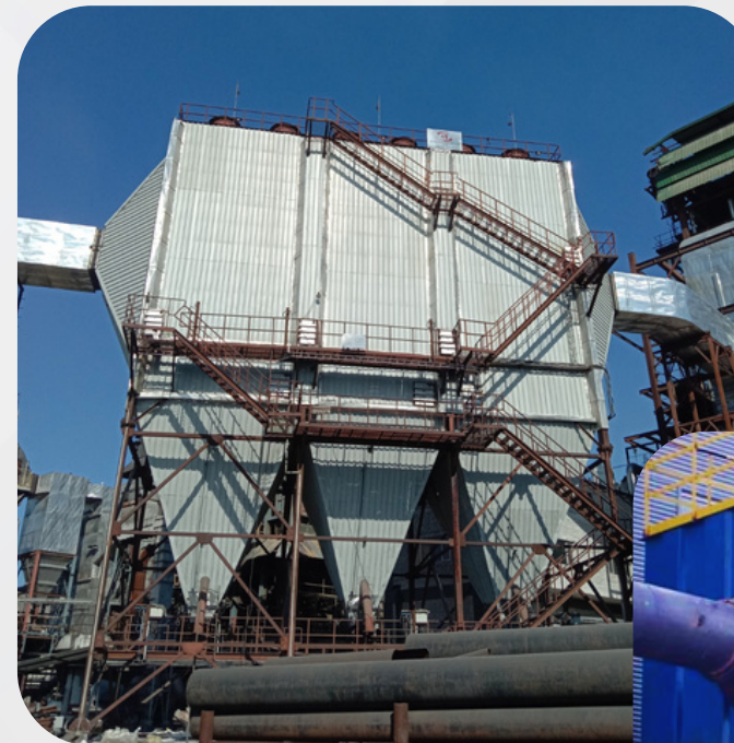
ELECTRO STATIC PRECIPITATORS
